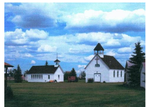
A Capital Improvement grant was awarded to the Flickertail Village near Stanley to re shingle several buildings in the museum complex.
