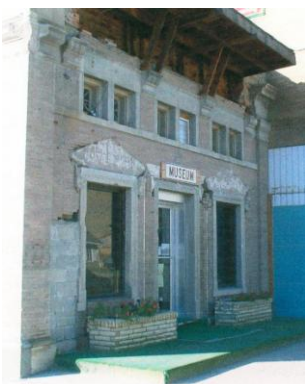
The Dickey County Museum received a grant to rehabilitate the front façade of the museum building.
